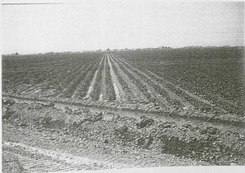
Plate C3.4 Individual Syphon Tubes from Earthen Header Ditch to Furrows
