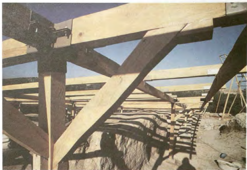
Photo 6 : The view of the construction system.
