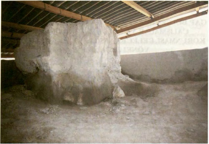
Photo 7 : Consolidation test of a mud-brick wall using a traditional techniques.
